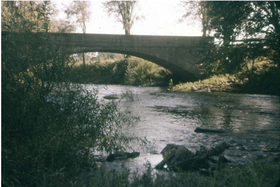
Allman Street Bridge Photo by Hildegard Kuse
