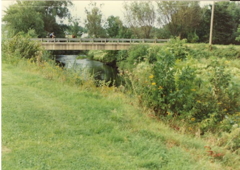
Bridge built in 1971 Photo by Loretta Kuse
