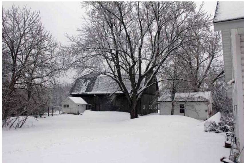
The Kuse Family Barn with a New Metal Roof – 2014
